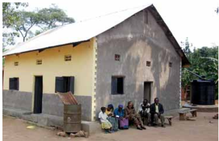
Sonia Mwadime and the Kaboggozas outside their renovated house. The water tank (right) was given to them by Biofresh
